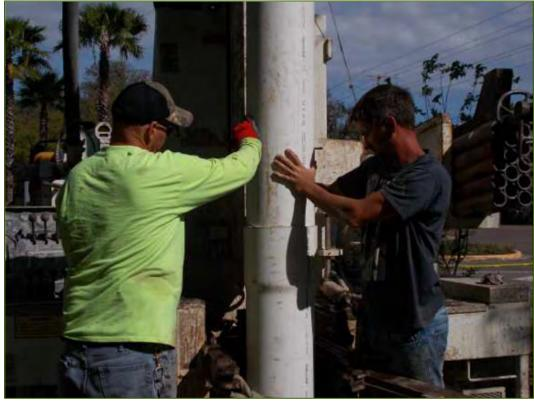
Photo #4. Grouting the Casing.
